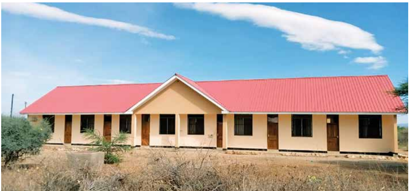
Picture 2: A six in one Multi-unit Teachers' House at Baray Secondary School in Karatu-Arusha.
